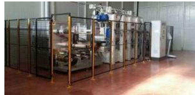
The new equipment for material fabrication installed on March 2018
